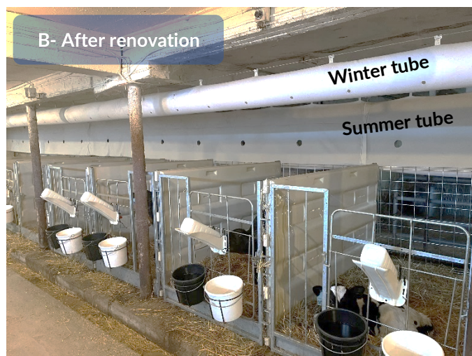
Figure 1. Renovating a 30-head tie-stall barn to house calves up to 8 weeks of age.
