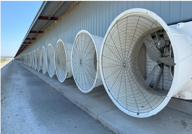
Figure 4. Keeping fans clean and functioning efficiently lowers energy costs and helps maintain consistent, effective ventilation throughout the barn. (photo: Aerica Bjurstrom)
