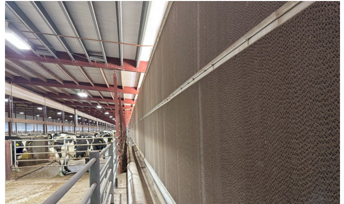
Figure 1. Evaporative cooling pads are installed at the air intake side of the barn and work by pulling air through a saturated medium. (photo: Aerica Bjurstrom)
